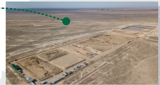
WMF Waste Management Facility
