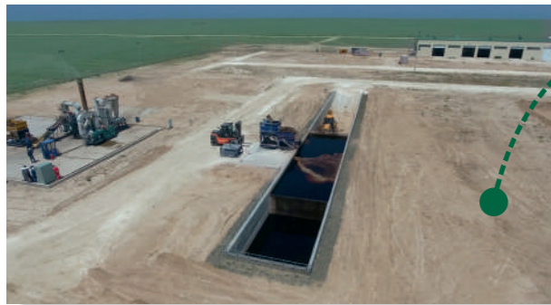
Koshanai Waste Management Facility
