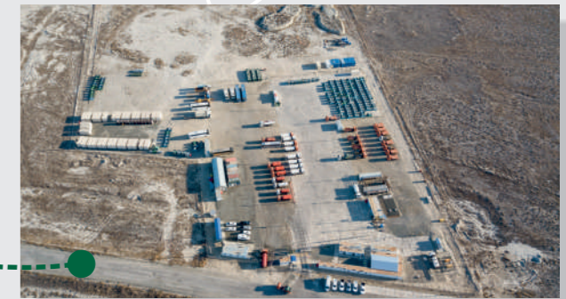
Tengiz Waste Management Facility
